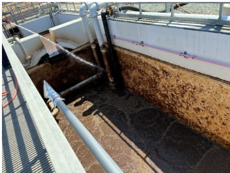
Aeration Basin #1 partially drained down
